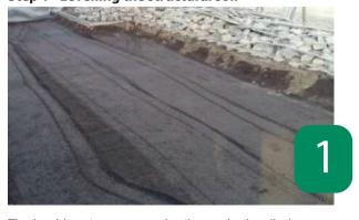
The load-bearing structural soil must be levelled.
