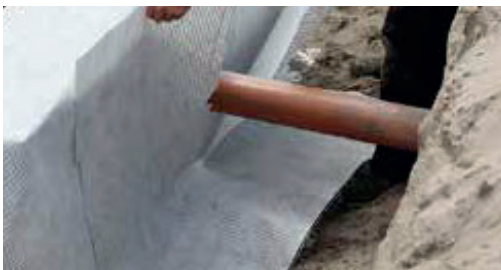
Use another piece of TP combigrid to make cover the cut. This cloth should overlap, 1m left and 1m right of the utility.
