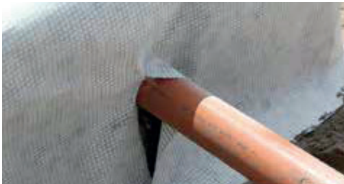
Make a straight cut in the TP combigrid around the TreeParker system up to the height of the utility.
