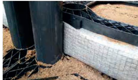
Use the TP combigrid to bridge the height in subbase material.
